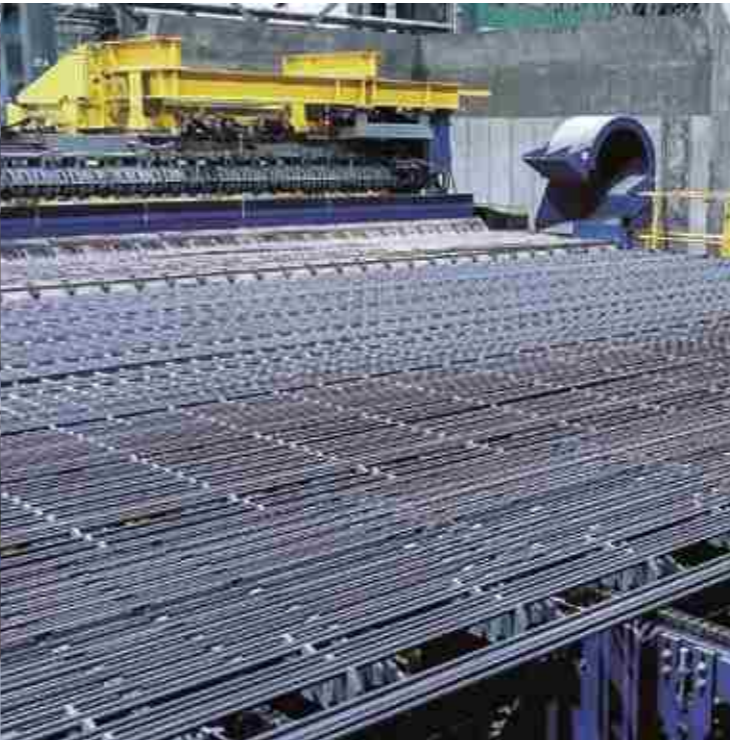
Cooling bed and bundling area
