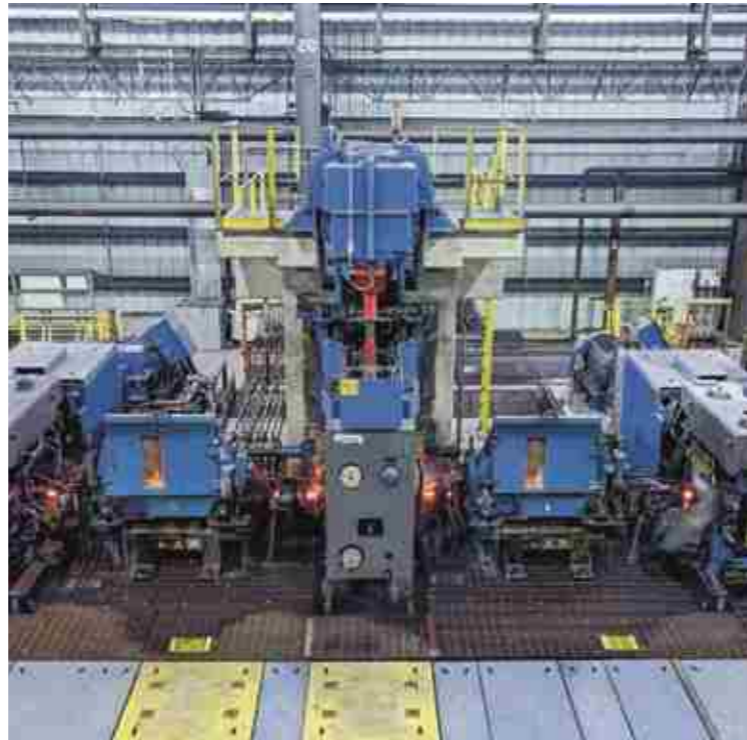
Housing-less stands on finishing mill
