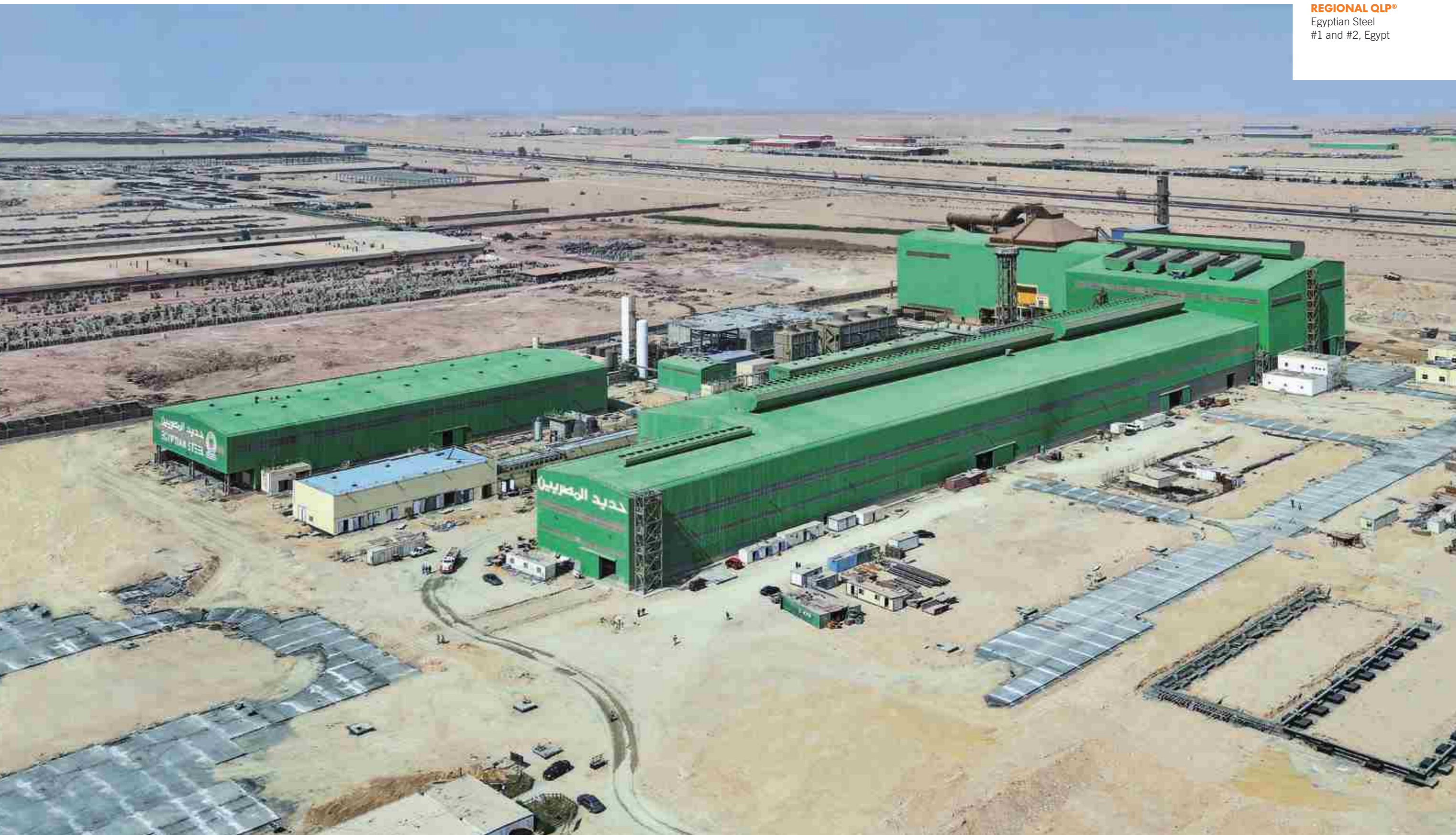
830,000 tpy MIDA QLP® minimill for rebar
