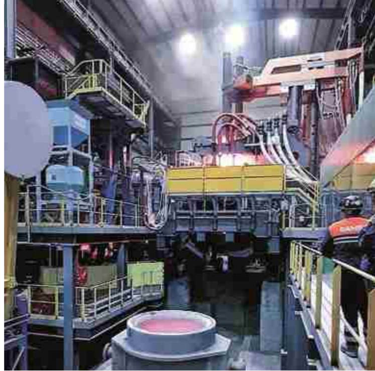
EAF meltshop continuously fed by preheated scrap through ECS®
